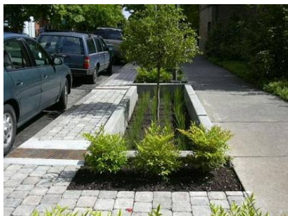
System of linked landscaped planters captures and attenuates surface water run-off. Planting within the structures adds visual interest and helps cool the air.
