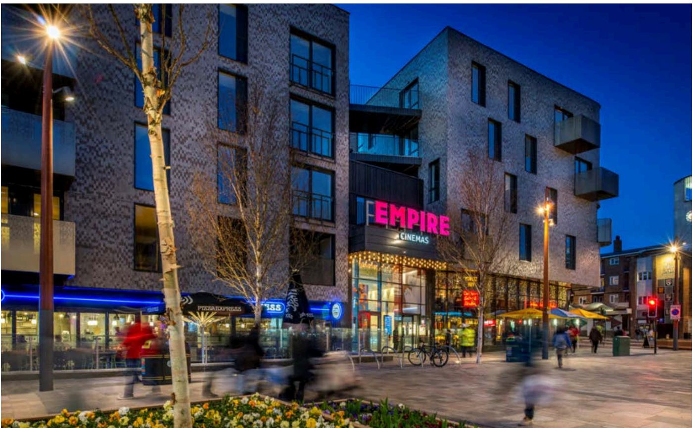
Homes can be incorporated over many other mixed uses to bring homes into the city. The Scene, Walthamstow, London. Pollard Thomas Edwards
